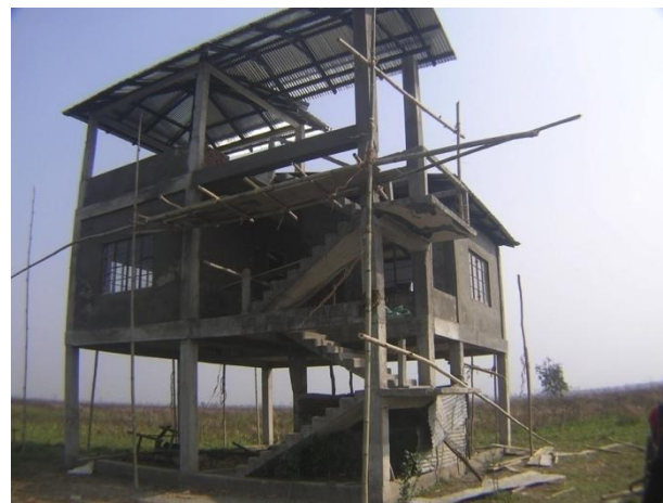
Figure 2. IRV 2020-funded infrastructure improvement in Manas National Park
